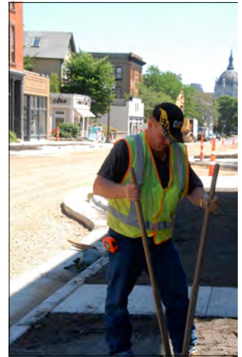
Construction foreman Gary digs the hole.
